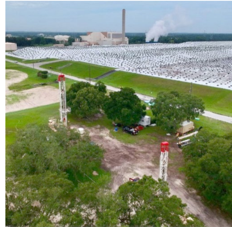
Pasco County Landfill Leachate Wells
